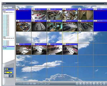
Central monitoring system up to 36 cameras
